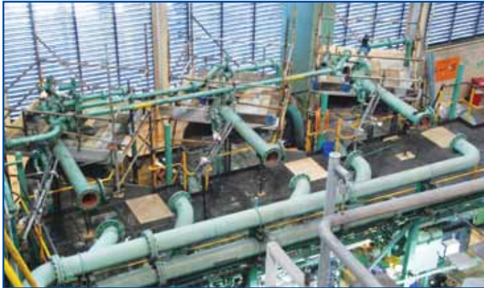
The polisher valves are being replaced as part of the overhaul.
