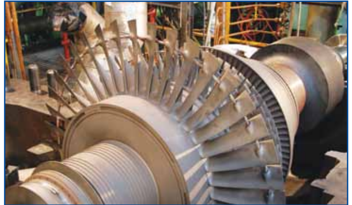
The steam feed pump turbine is currently being overhauled by Siemens.
