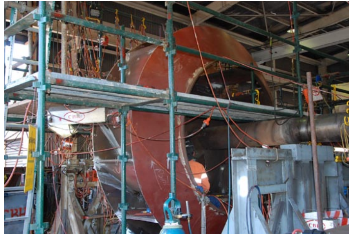
Replacement of the ID fan impellers will begin in mid February.
