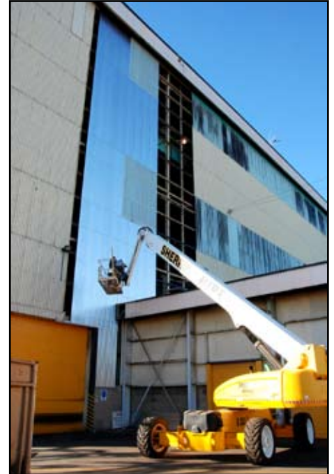
Wall sheeting almost complete.
