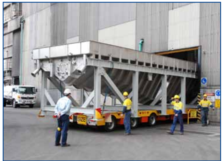
...And in with the new ash hopper
