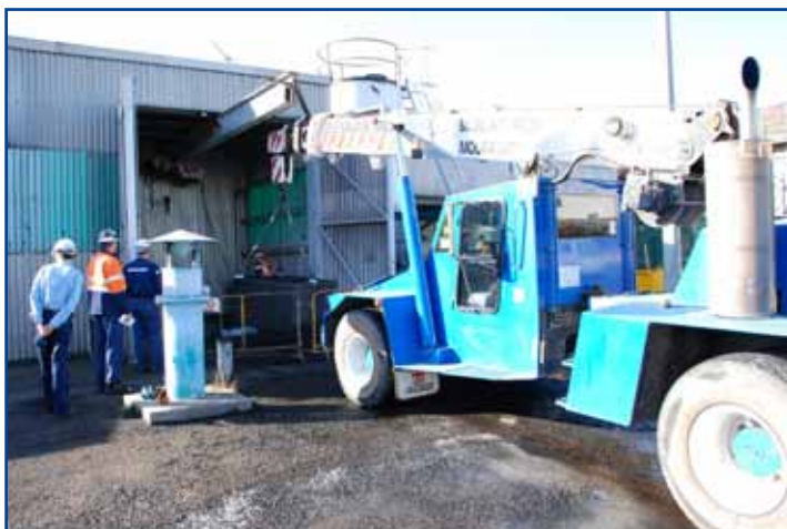
A magnet from the coal unloading facility is taken away for refurbishment.
