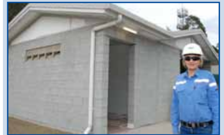
Local contractor Jayne Marshall checks out the new ladies toilet.
