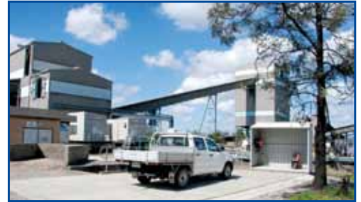
New car wash facility
