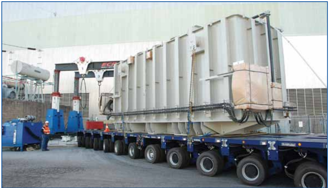
The 168 tonne transformer is transferred to the purpose built storage bay.
