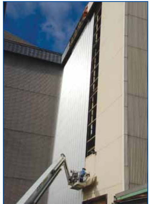
EB Plumbing complete work on turbine hall wall sheeting.
