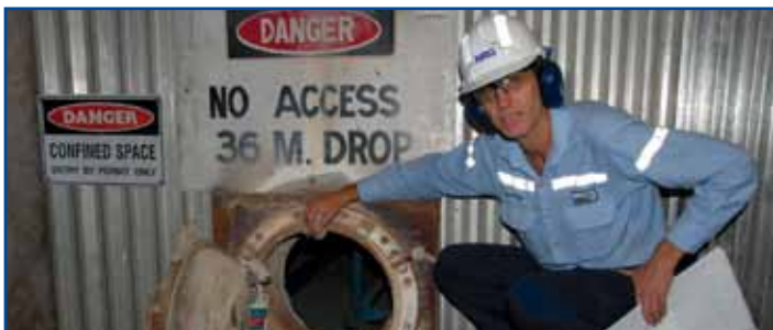
Dave Greinke inspects the old entry point to the boiler furnace.
