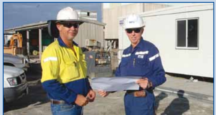
Stewart and Rick check out plans for the new Dodds Construction facility.
