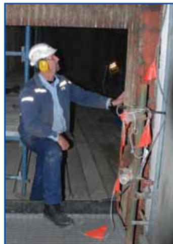
Graeme Hawke checks out the expanded entry to the boiler furnace.
