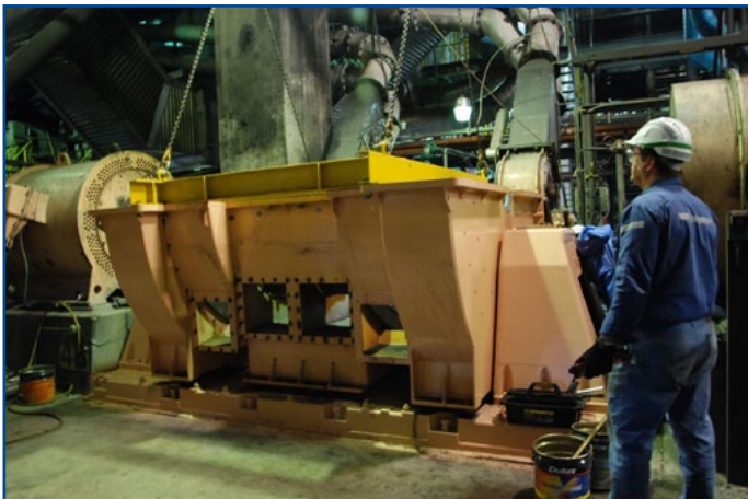
Ron Williams lowers the pulveriser case into position.
