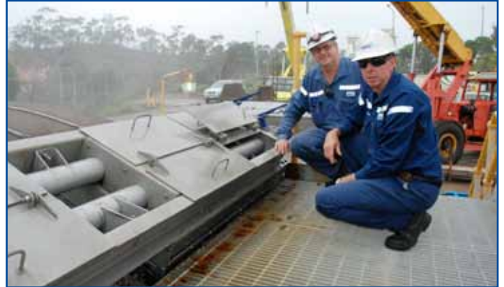
Neil Grother and Rick Thomason check out the new spray boxes on the CW screens.
