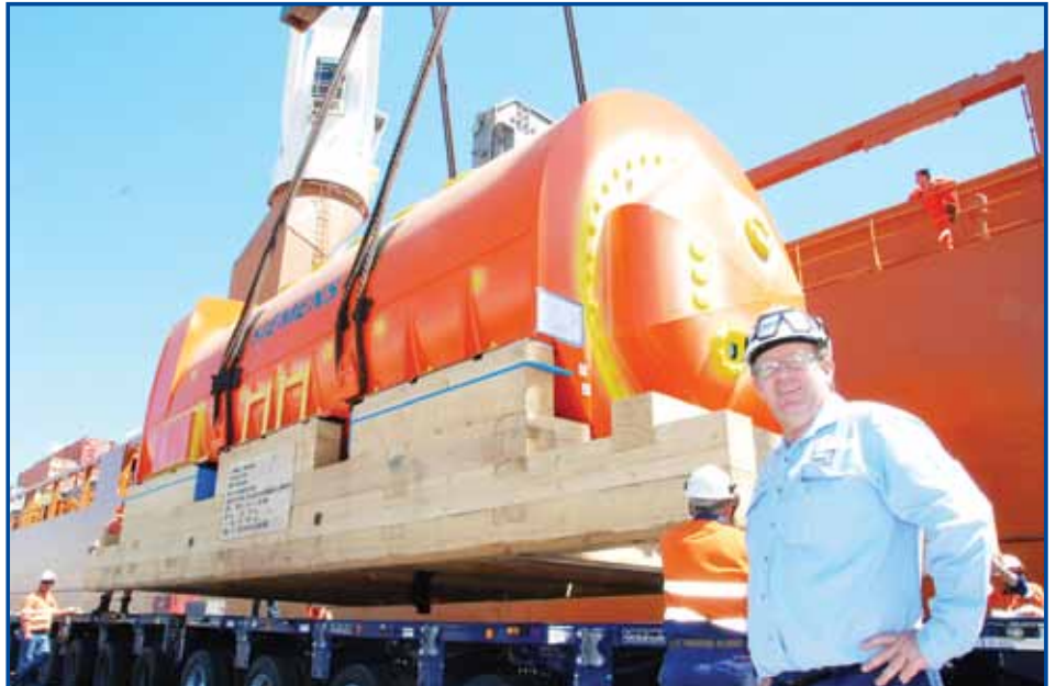
Manager Major Projects, Steve Lewis was on hand to inspect the new generator that arrived at Auckland Point wharf last month.
