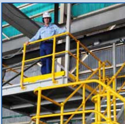
Dave Greinke checks out the safe access platform used to access the service floor hoists.
