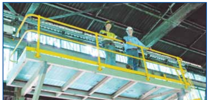
Dean Marsh (Walz Construction) and Graham Long inspect one of the new platforms in the slot bunker which will allow for easy maintenance of the cranes.
