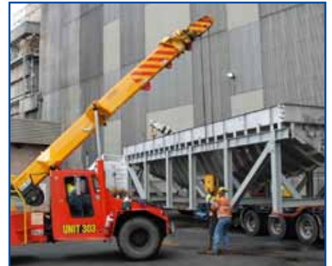
The new Unit 3 ash hopper arrives.
