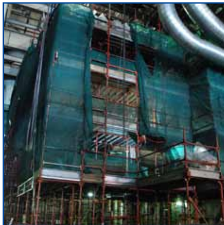
The round flue duct cladding project access scaffold.
