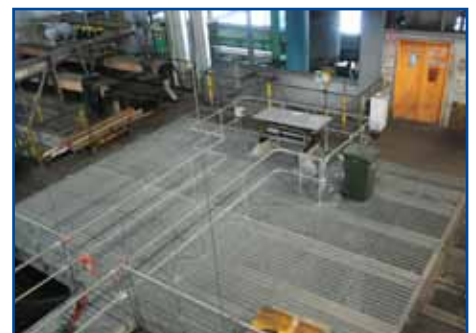
The new winching area installed for the overhaul.
