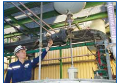
Ross inspects part of the demin plant which is being refurbished.
